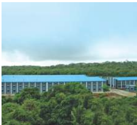
DG Set Manufacturing Unit Kalsar, Gujarat
